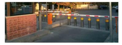
This is an integrated Electro-Hydraulic Rising Bollard. This equipment is mainly used to control the vehicle access. It can work together with the parking barrier system or work as standalone. This machine is designed and developed to prevent un-authorized vehicle forced entry into sensitive area. There arects are widely used in Urban trans-
